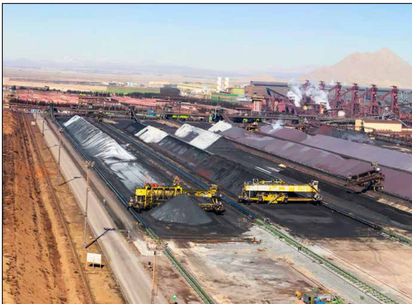
1- High pressure grinding rolls
